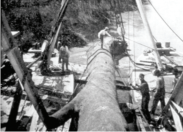
Figure 5. An early photograph of snag removal in the Mississippi River. Snag removal conducted in concert with sandbar dredging represents the earliest attempts to improve navigation on the Upper Mississippi River and served as a precursor to more highly engineered channel development measures. Improved navigability lead to expanded floodplain development and sequestration of floodplain environments from the main channel of the river. (Photograph from N. Moore [1972].)
