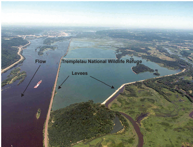
Figure 4. An example of the effects of levee construction on lateral connectivity by Trempeleau National Wildlife Refuge, Wisconsin. This aerial photograph demonstrates the lack of hydrologic connectivity that exists following levee development. Water in the Mississippi River ( left side of photo) is clearly darker than water on the refuge side of the levees, suggesting no hydrologic mixing. Correspondingly, water, nutrient, energy, and biotic exchange between the main channel and the floodplain are severed.
